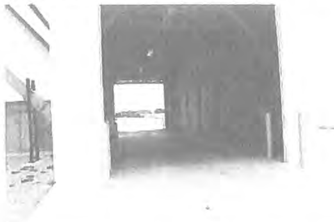
View of what the future tractor trailer unloading building (OC-2) adjacent to dry fertilizer building will look like when completed
