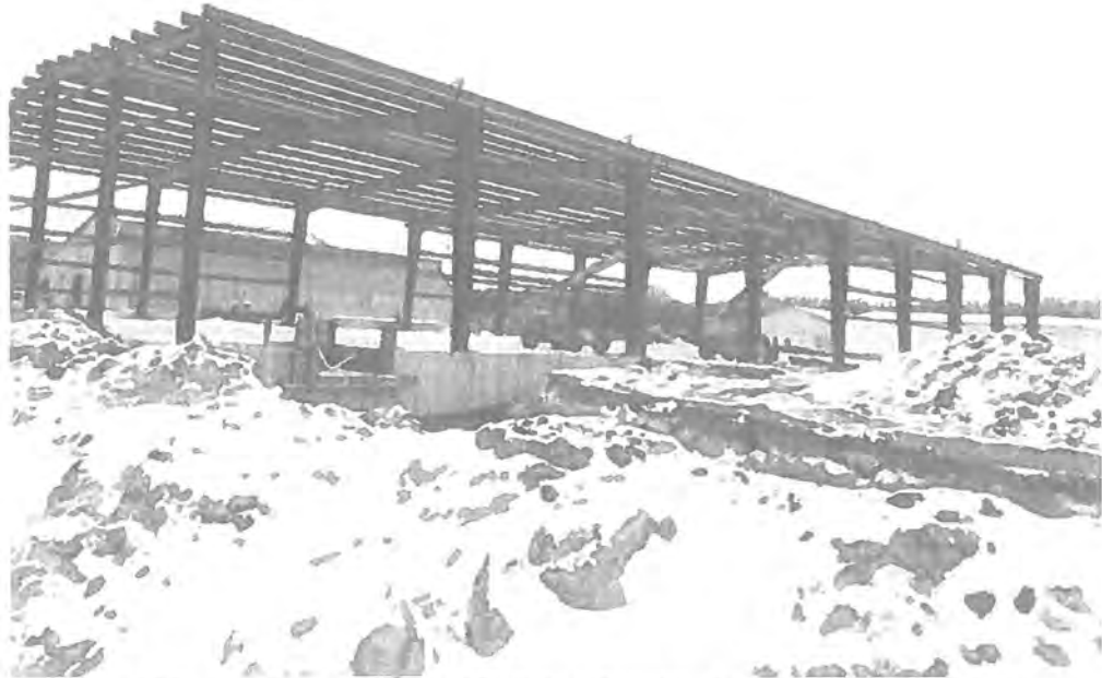
Liquid Fertilizer and Chemical Building Construction as of 12/20/2022
